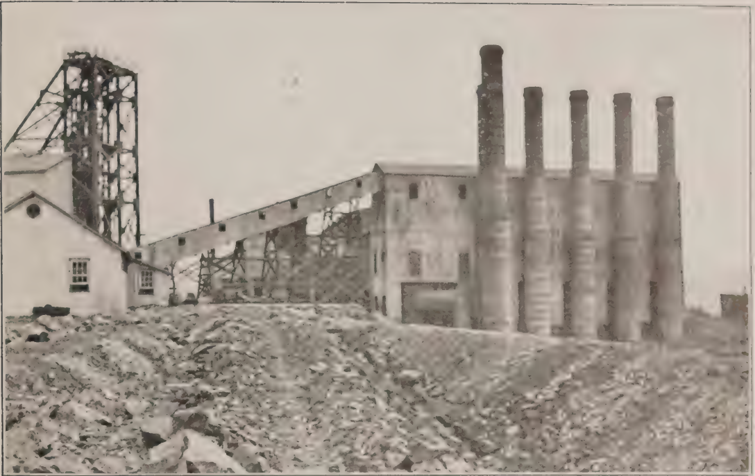
Magpie mine: head frame and roaster stacks.
